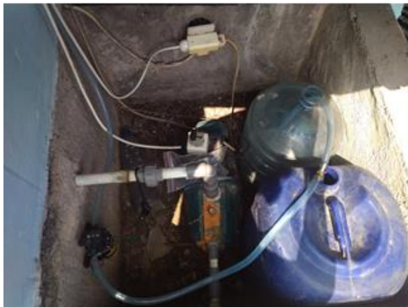
Figure 6. Installation of pumps, power, and disinfectant fluids
